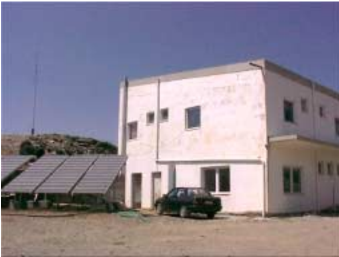
Figure 8: PV – system module 2 with appartement house
