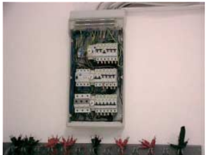
Figure 18: Sub-distribution for the electrical station
