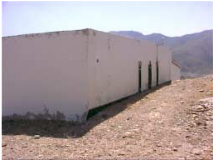
Figure 11: Electrical station (backside) with entrance of cables and wires
