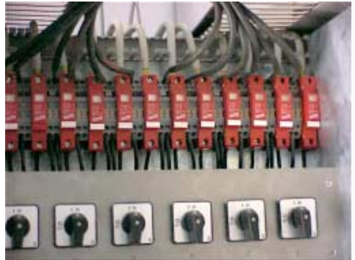
Figure 14 : Available SPDs for the PV-systems 1 and 2
