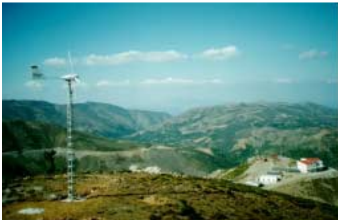
Figure 1: Top view of the hybrid-system VATALI location
