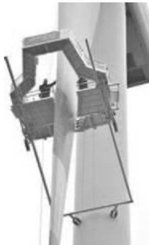
Figure 1: Conventional climbing frame for WTB [2]
