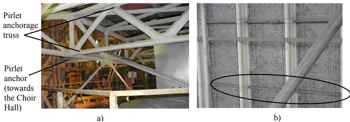
Figure 3. Anchorage truss at the Octagon (a) and Anchors around the Choir Hall (b).
