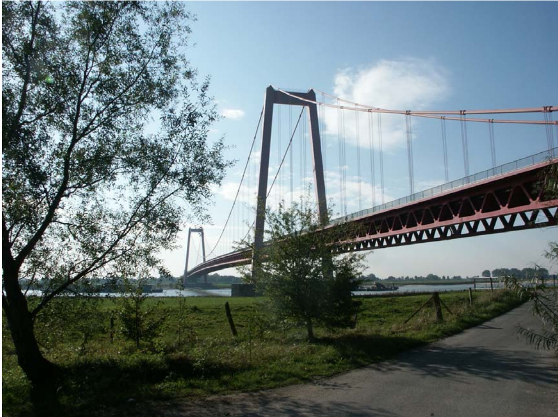
Figure 4: Rhine bridge Emmerich
